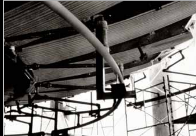
Clamp-on PLATECOIL attached to large butane storage tank
